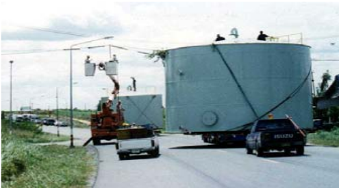
Road modification for two oversized tanks
