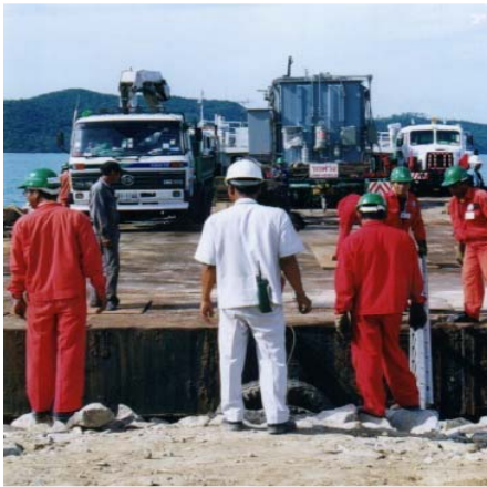
Preparing an “artificial jetty” at Samui Island to discharge the 2x98-ton Transformers
