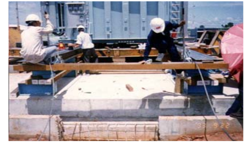
Skidding transformer using winches
