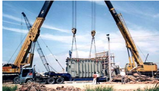
Offloading in a remote area with a 80-ton and a 50-ton mobile crane
