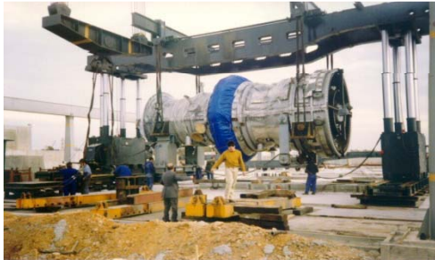
Using 600-ton modular hydraulic gantry crane
