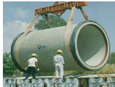
Loading coated pipes with soft slings to protect their coating
