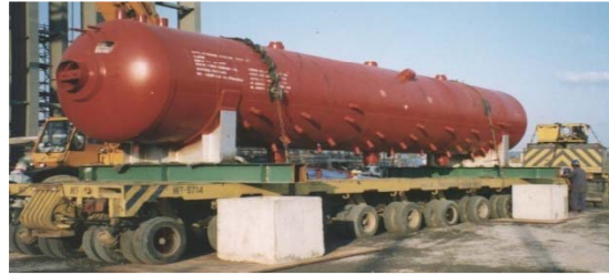
A 120-ton boiler upon delivery to jobsite
