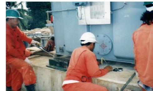
Fine tuning and positioning the transformer
