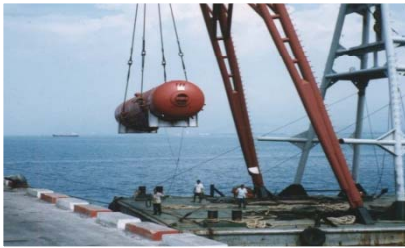
Discharge a 120-ton boiler with floating crane
