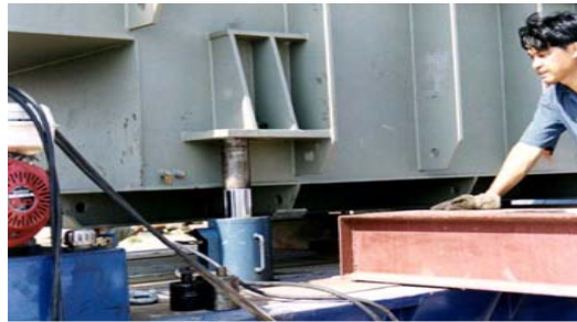
Placing the hydraulic jacks and inserting the skid beams
